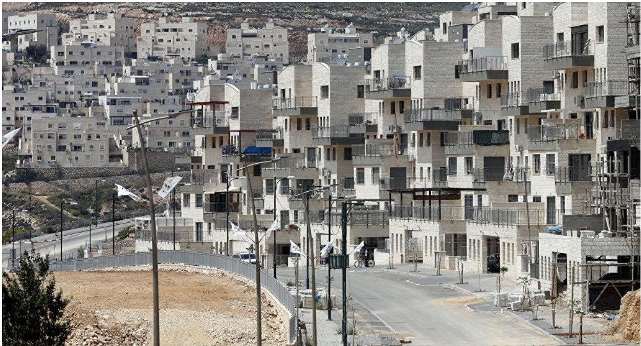
Illegal settlement homes
